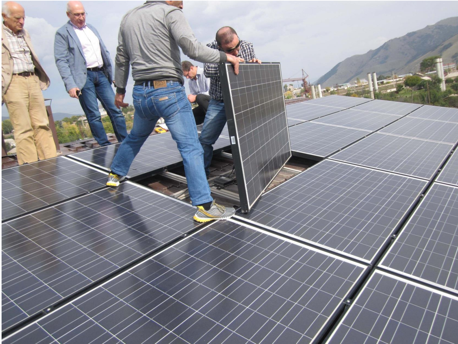
17 KW PV station installed at the roof of YMCA building in Spitak, October 06, 2015
